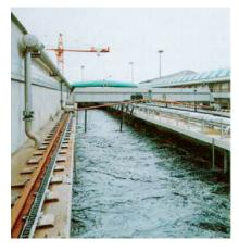
Fig. 8.63. By injecting  $FeCl_3$  into the sludge, dissolved phosphate precipitates from the waste water
